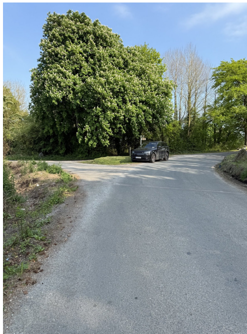
The bend. Disturbed verge on the left. The turn she had to make is ahead. No cone in this frame.
